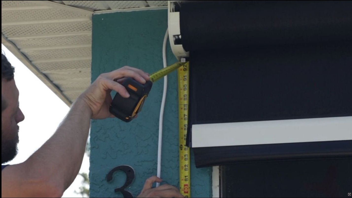
Measuring tacks before cutting tracks
