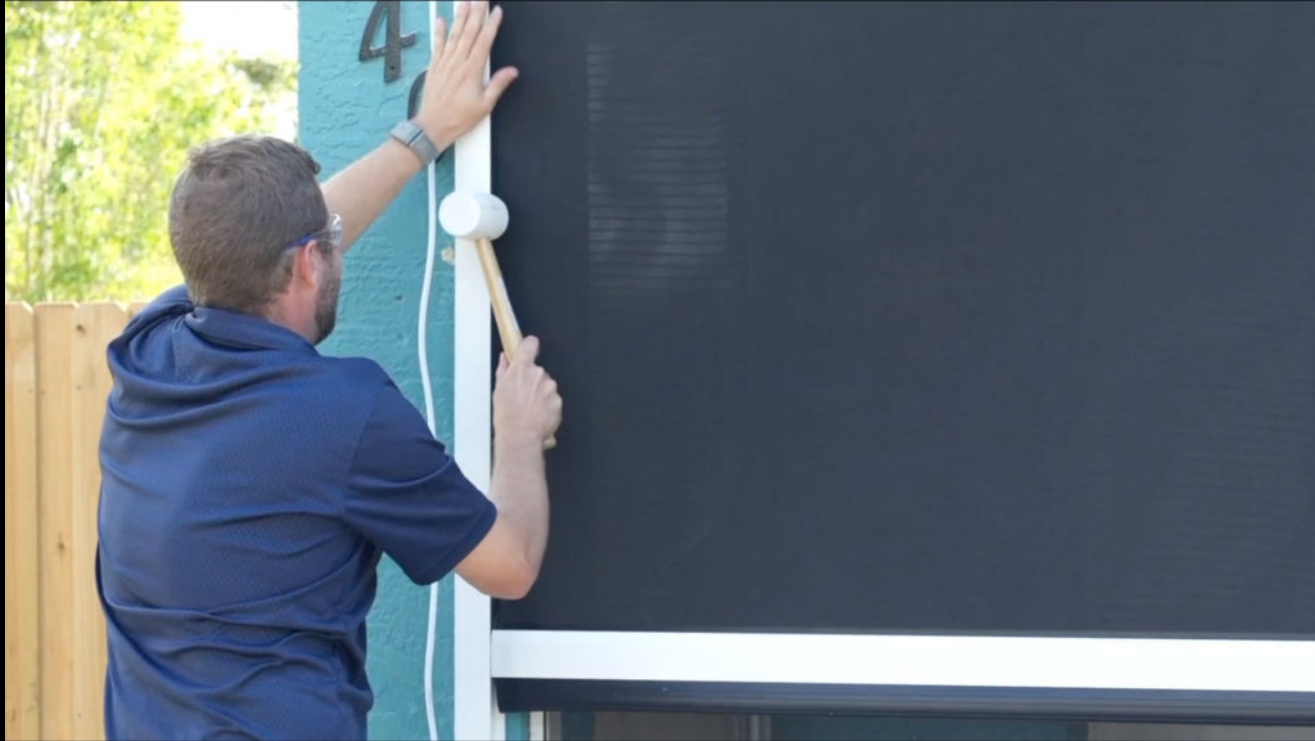
Attach track covers using rubber mallet
