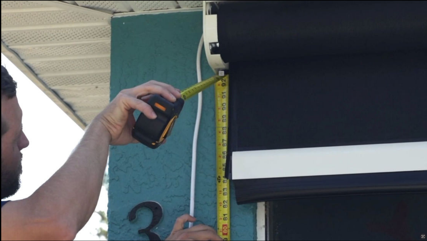
Raise screen to temporary upper limit. Measure for the tracks from ground to bottom of housing
